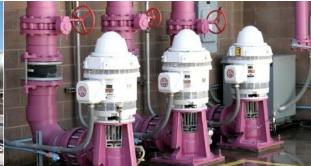
Automated Asset Management
