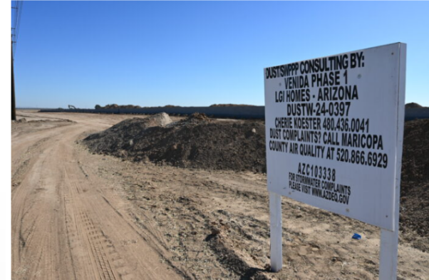
Construction at Venida 1 on Papago Road photographed Dec. 2, 2024. [Jeff Chew]
