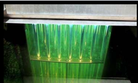
Advanced water treatment systems
